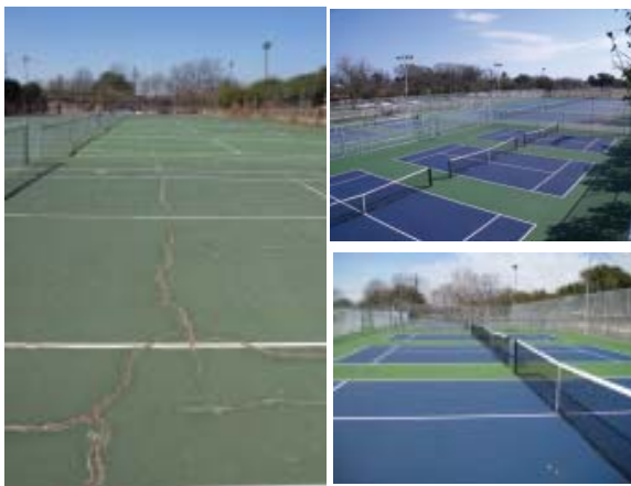
Kiest Park Tennis Courts - Before & After the Renovation
